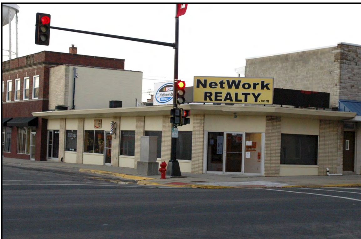
View of the resource, looking southwest across the intersection of 1 st Ave. W. and W. 2 nd St. S. The narrow two-story section at the south end of this building houses the stairway to the second floor of the brown brick building at 109-111 W. 2 nd Street S.
