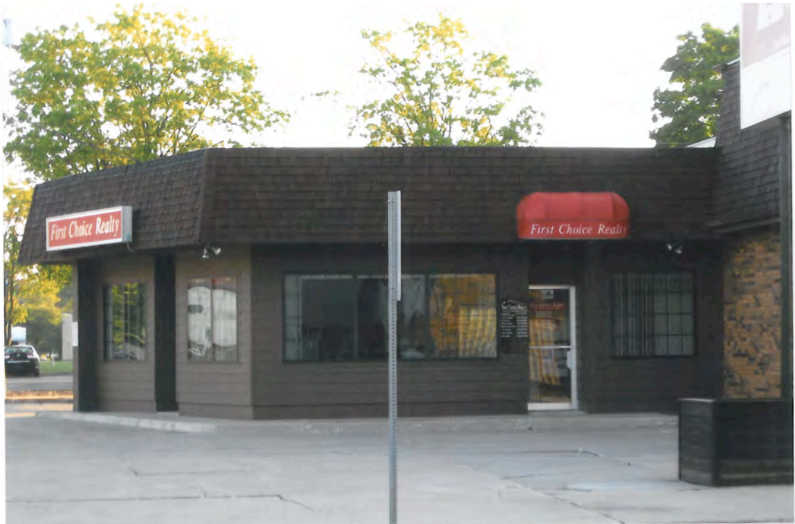
This is the only portion of the 1963 service station still visible. It was the station office.
