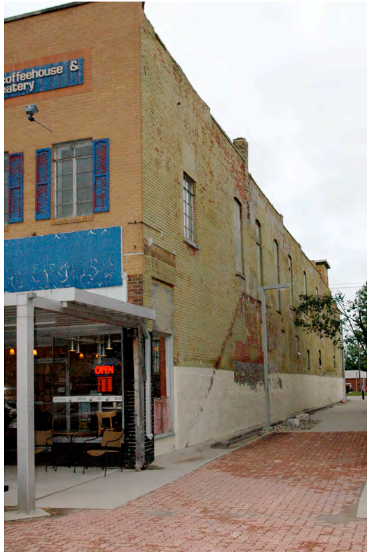
View of the east (alley side) elevation, looking northwest.
