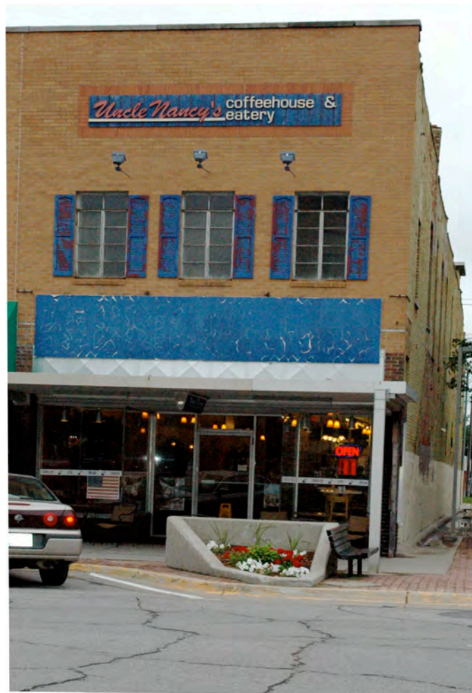
View of the resource, looking north across N. 2 nd Avenue W.
