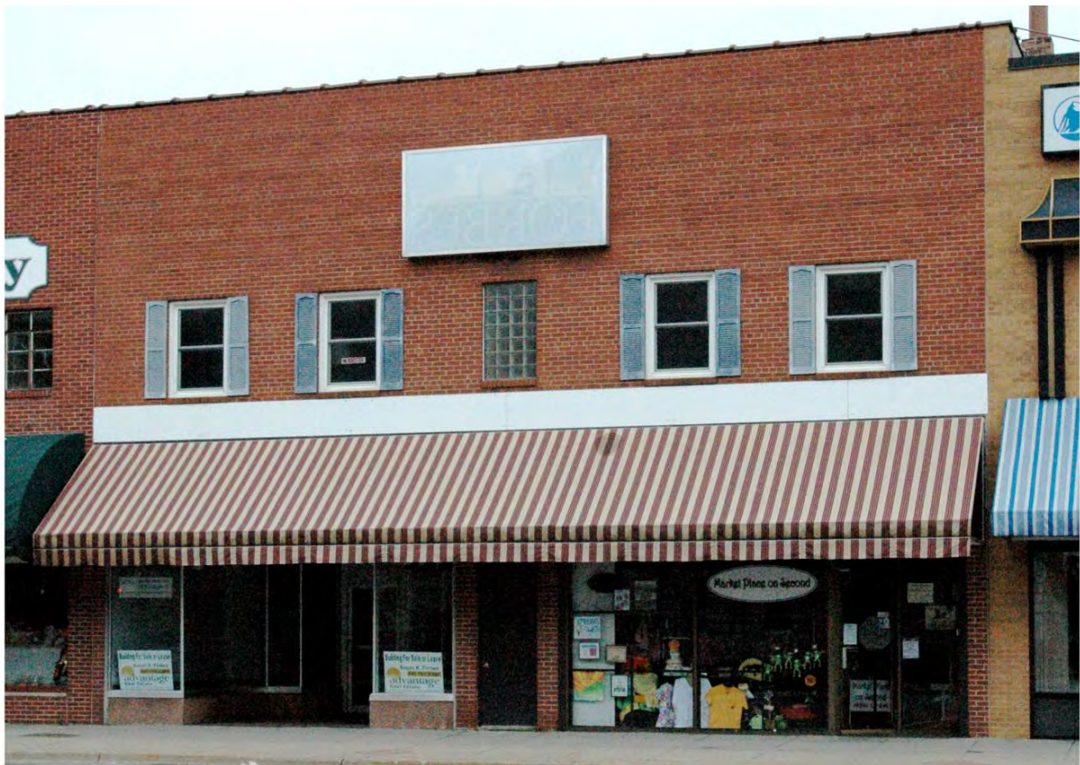
View of the resource looking west across W. 2 nd St. N.
